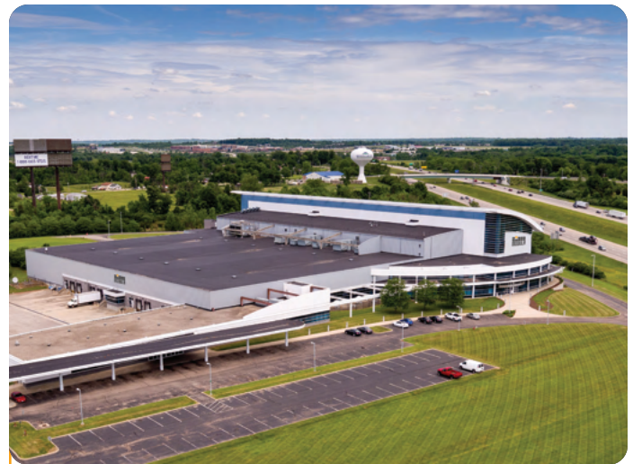
Modula Plant – Franklin, Ohio
