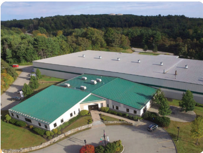
Modula Headquarters and Plant – Lewiston, Maine
